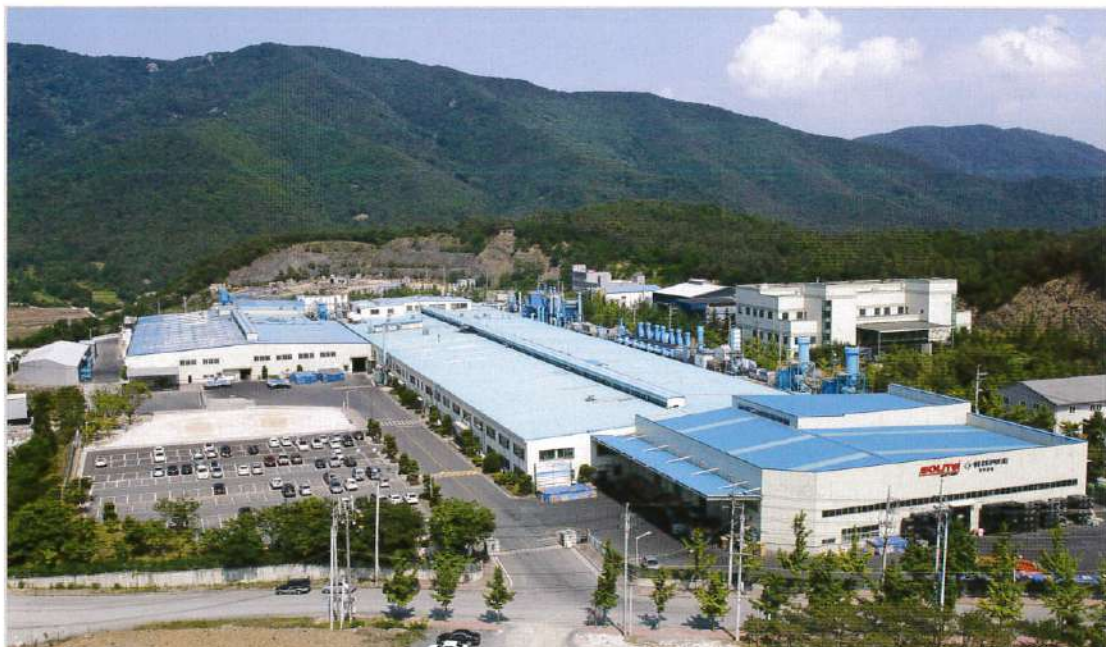
Battery Plant in Gyeongju
